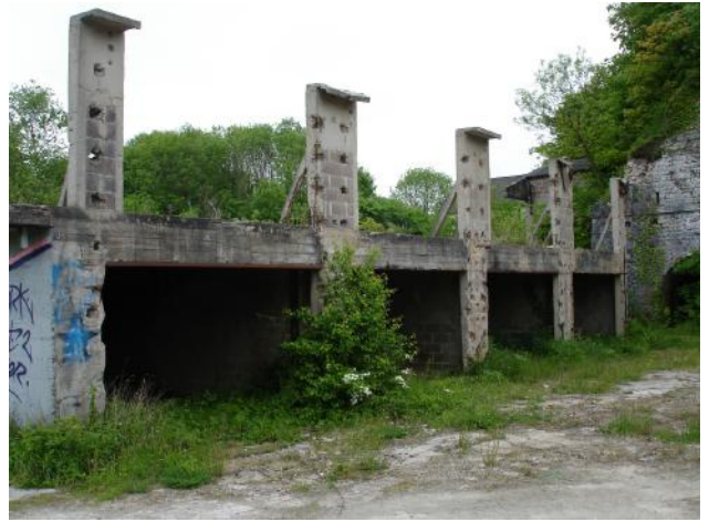
Hangar, Roque Genest
